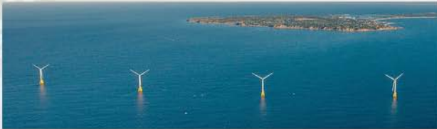
The first offshore wind power plant in the US, with the capacity of 30 MW (Photo courtesy of General Electric (GE), Inc.)
