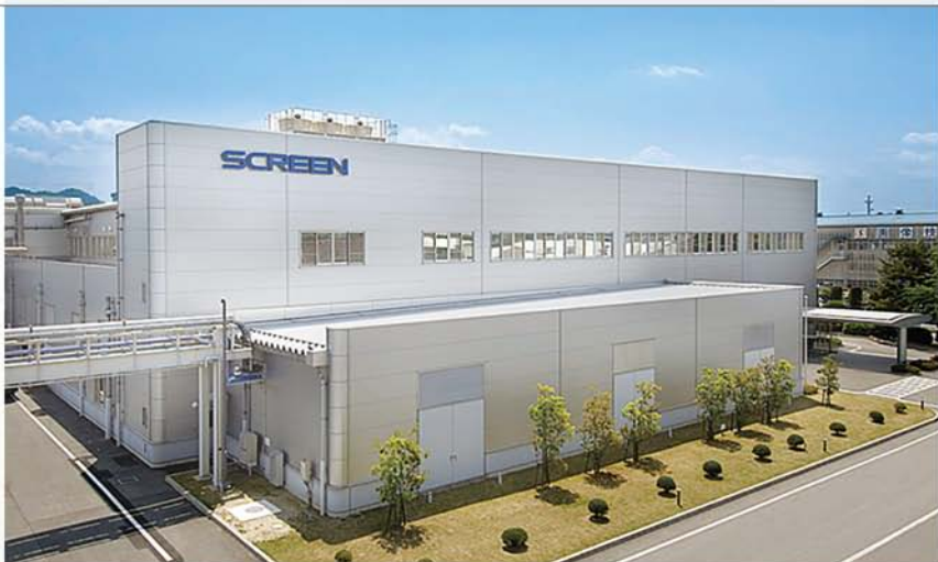
SCREEN Semiconductor Solutions' fabrication plant in Hikone, Japan (Photo courtesy of SCREEN SPE Taiwan Co., Ltd.)
