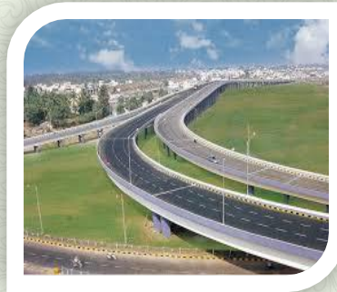
Construction of Road, Bridge and Railway Line
