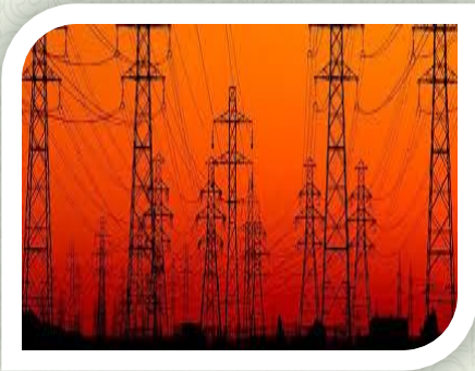
Power Generation, Transmission and Distribution
