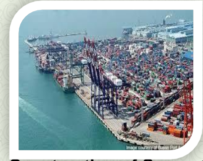
Construction of Seaport, River Port and Dry Port
