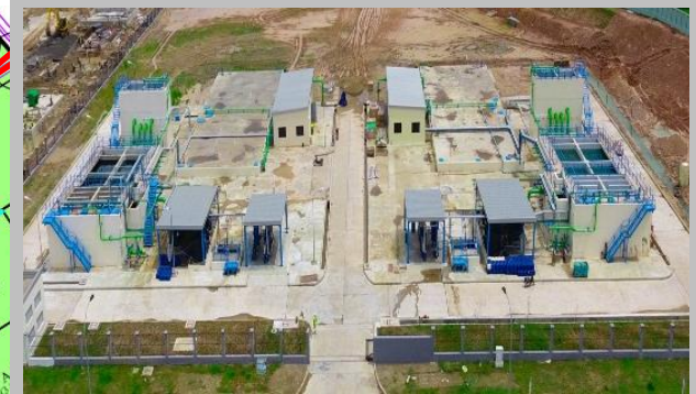
(1) Water Purification Plant [Present Capacity; 6,000m 3 /day]
