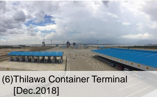
(6) Thilawa Container Terminal [Dec.2018]
