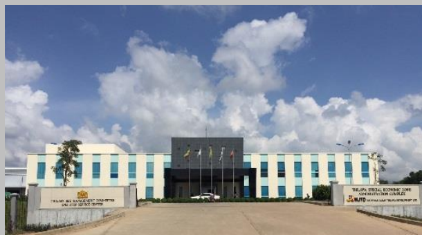
(3) SEZ Administration Building [MJTD, TSMC, Banks, Insurance Companies Office]
