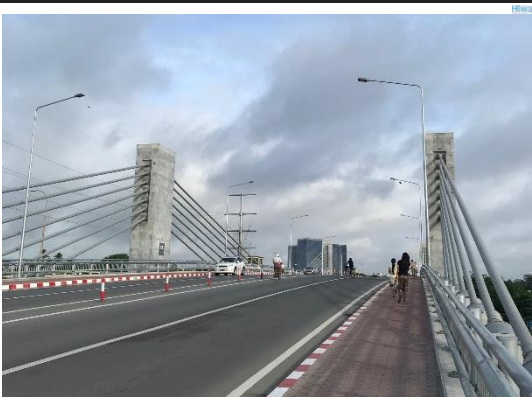
(8) Thaketa Bridge [Jun.2018] (9) Bago Bridge [Year 2022] (10) Thanlyin-Thilawa Road [Jun.2019]
