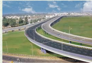
Construction of Road, Bridge and Railway Line
