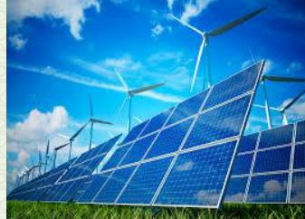
Production of Renewable Energy
